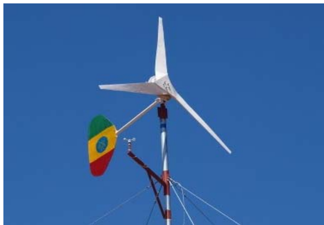
Fig. 6. The 3m rotor diameter LMSWT installed at the rural community of Handew in the Somali region of Ethiopia
